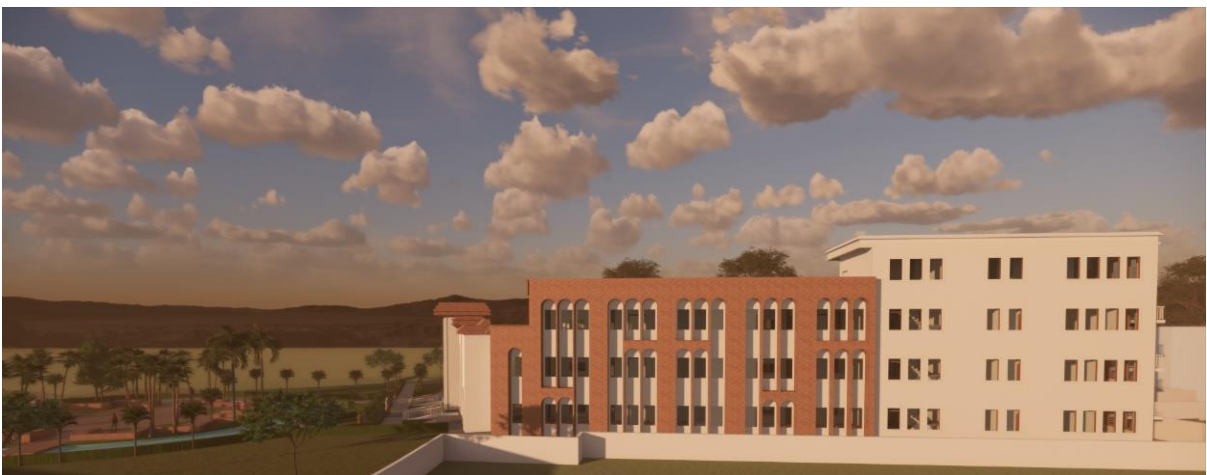
Figure 12: Building from Western Side
